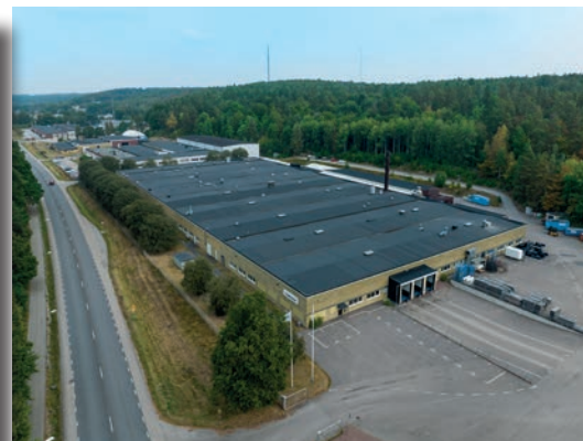
Safeman AB - Olofström, Sweden Building area: 13.000 m 2 (owned)
